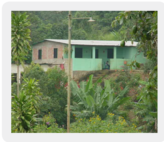
Figure 1: El Paulino typical construction
